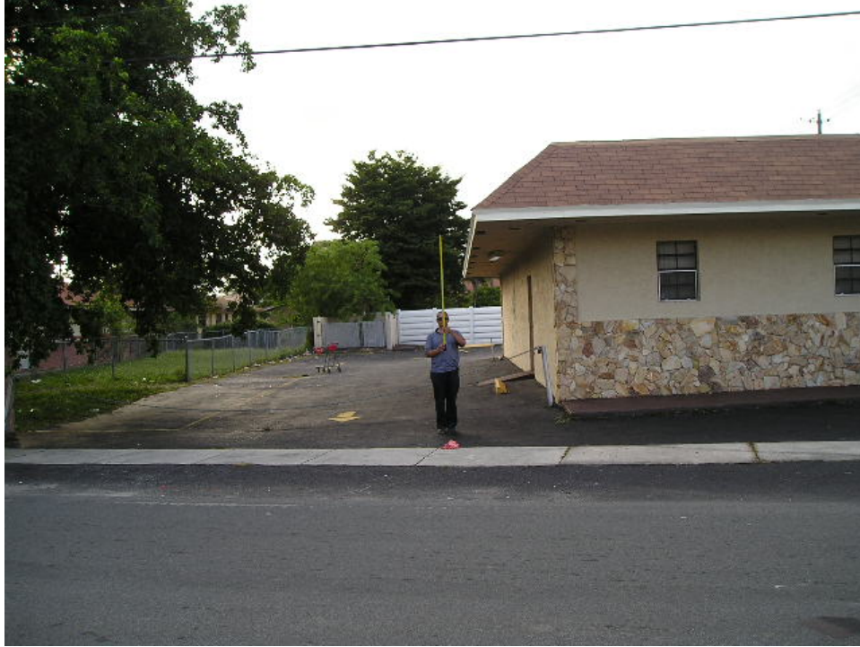
1. VIEW WESTERLY ALONG NORTH BOUNDARY OF SUBJECT PROPERTY (showing proximity of adjacent building roofline) FROM ACROSS NW 7AVE.
