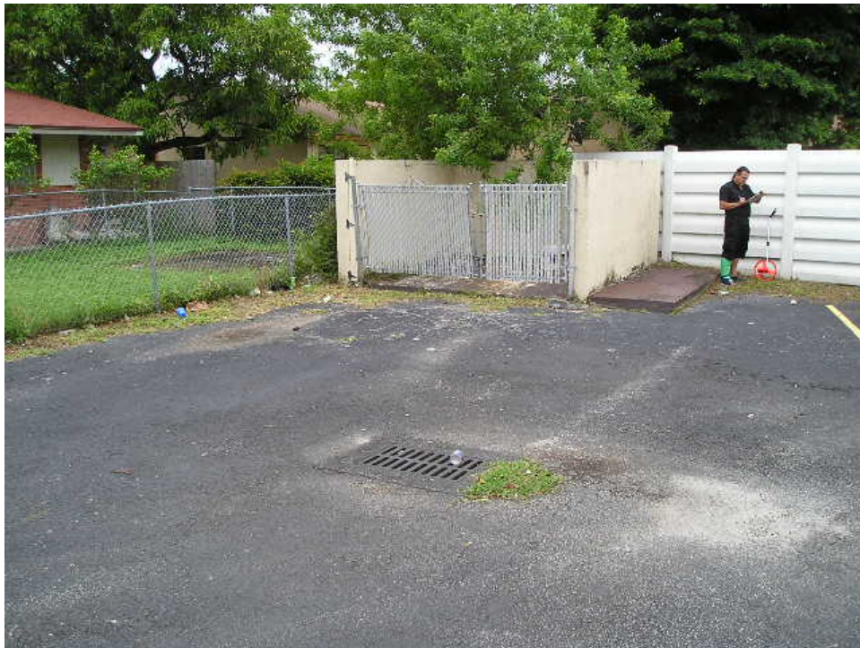
6. VIEW SOUTHWESTERLY OF DUMPSTER ENCLOSURE, PAVING, CATCH BASIN AND CONCRETE FENCING (only asphalt paving is included in valuation)
