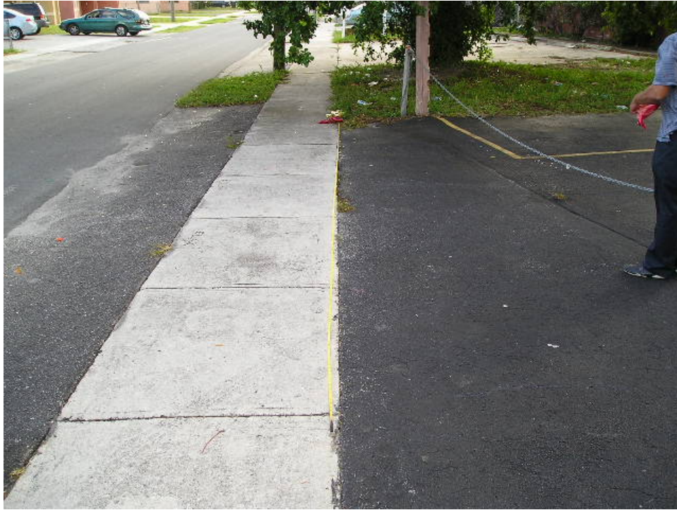
3. VIEW SOUTHERLY ALONG EASTERN PROPERTY BOUNDARY (back of walk)
